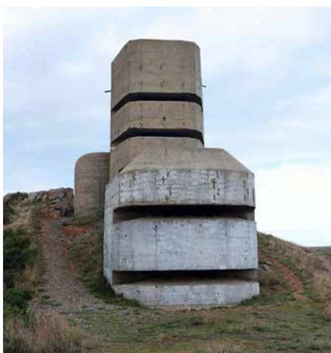
The unusual offset design of MP4 is unique. It served the same purpose as the round range-finding towers. Built on five levels, each level was to have served one of the five naval gun batteries planned for the island. In the event only three naval batteries arrived, and the two other levels were used by the army. In the latter part of the war a Freya radar was mounted on the roof
